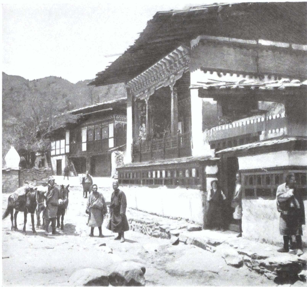
Wooden houses, with wooden roofs in the form of planks, kept from blowing off by large stones. 2
